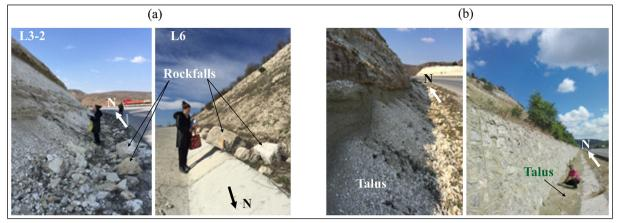
Figure 3- Geotechnical problems due to undercutting processes; a) rockfalls and b) the filling of road drainage ditches (Kütahya-- Eskişehir road, Ilica location).
