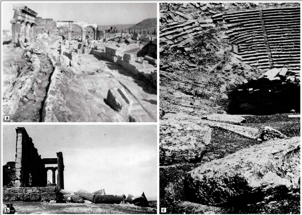
Figure 6- a) Photo presented in D'Andria et al. (2008) showing the deformations that occurred during the 7 th century earthquake on the Plateia (city square) extending to the Frontino Gate, which was taken during the 1963 excavations in Hierapolis. Some photos in Rudolf Naumann's work documenting damage after the March 28, 1970 Gediz Earthquake in the ancient city of Aizanoi; b) systematic aligned fallen columns of the Temple of Zeus, c) deformations in the cavea of Theater and lateral displacements in large buried marble blocks.
